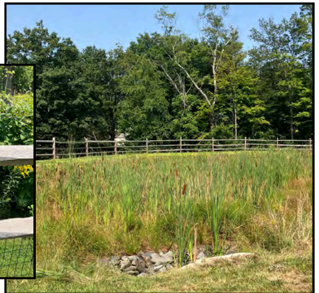
Stormwater basin in Dallas Township designed to empty within 72 hours so it doesn't serve as a mosquito breeding site
